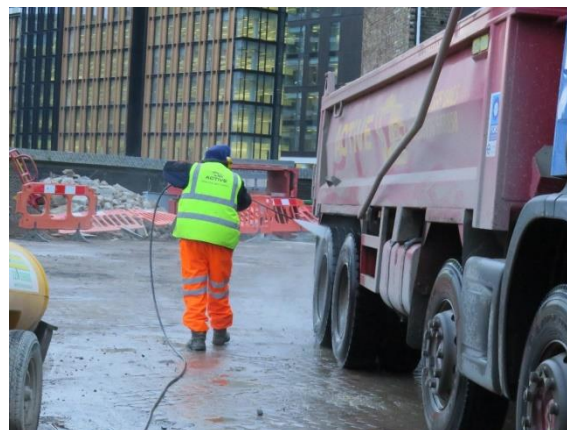
Figure 11 Wheel washing to reduce material tracked out of the site
